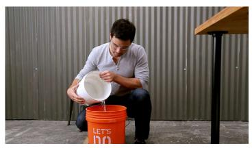
Put 3 inches of concrete mix in the bucket. Make sure the bucket is clean and dry before opening up the concrete and scooping 3 inches of concrete mix into the bucket. Add some water and start mixing. Be careful not to over water the concrete or it will be weak and crumble. Thoroughly mix the concrete so that every grain of the mix is wet. The mix should be the consistency of cookie dough.
