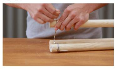
Insert wire. Insert the wire into the holes you just drilled and wire the 3 legs together. The wire keeps the legs from coming our of the concrete.
